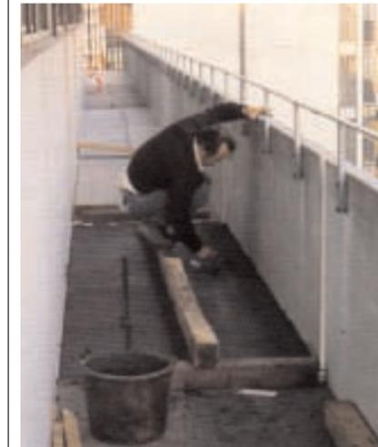
Figure 6. Renovation of balcony walkway with Densitop®.
